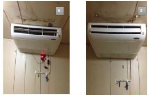
Cool room with Coolbot (A) and cool room with local modification (B)
