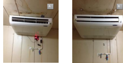
Cool room with Coolbot (A) and cool room with local modification (B)
