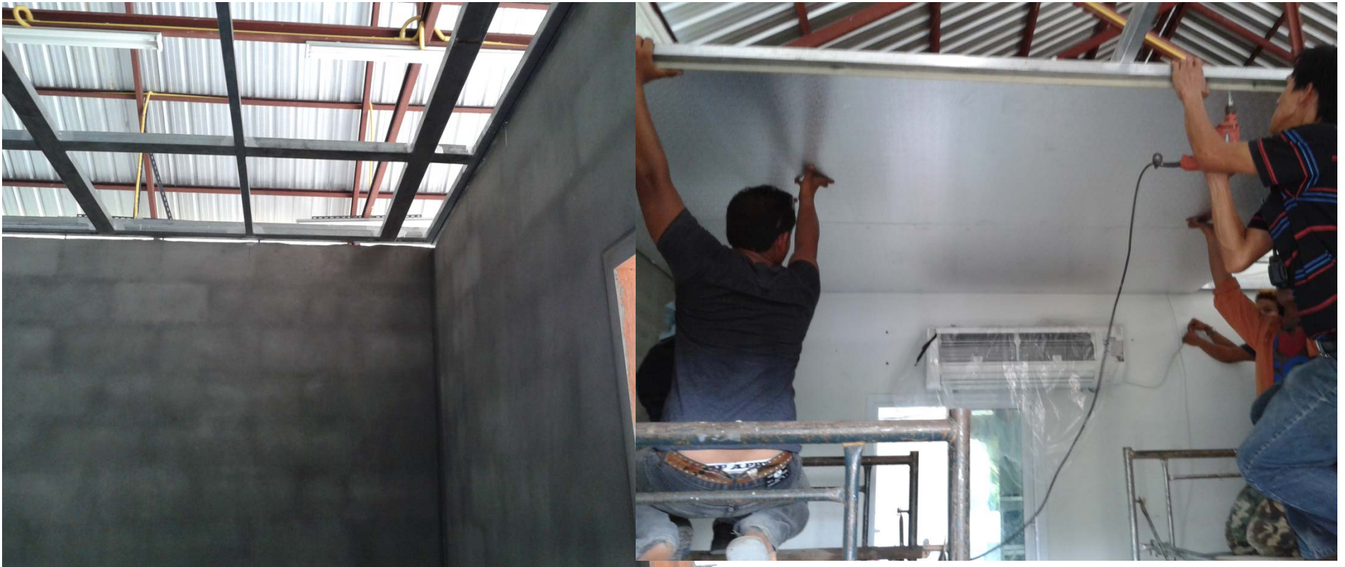
One inch polyurethane insulation
