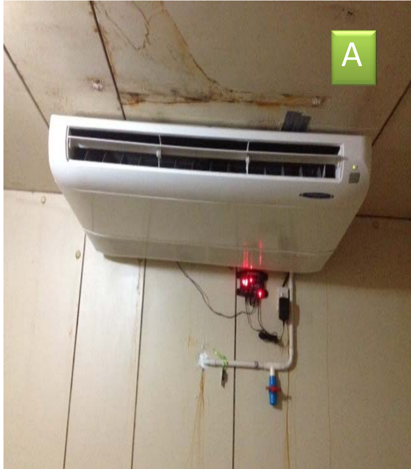
Cool room with Coolbot (A) and cool room with local modification (B)
